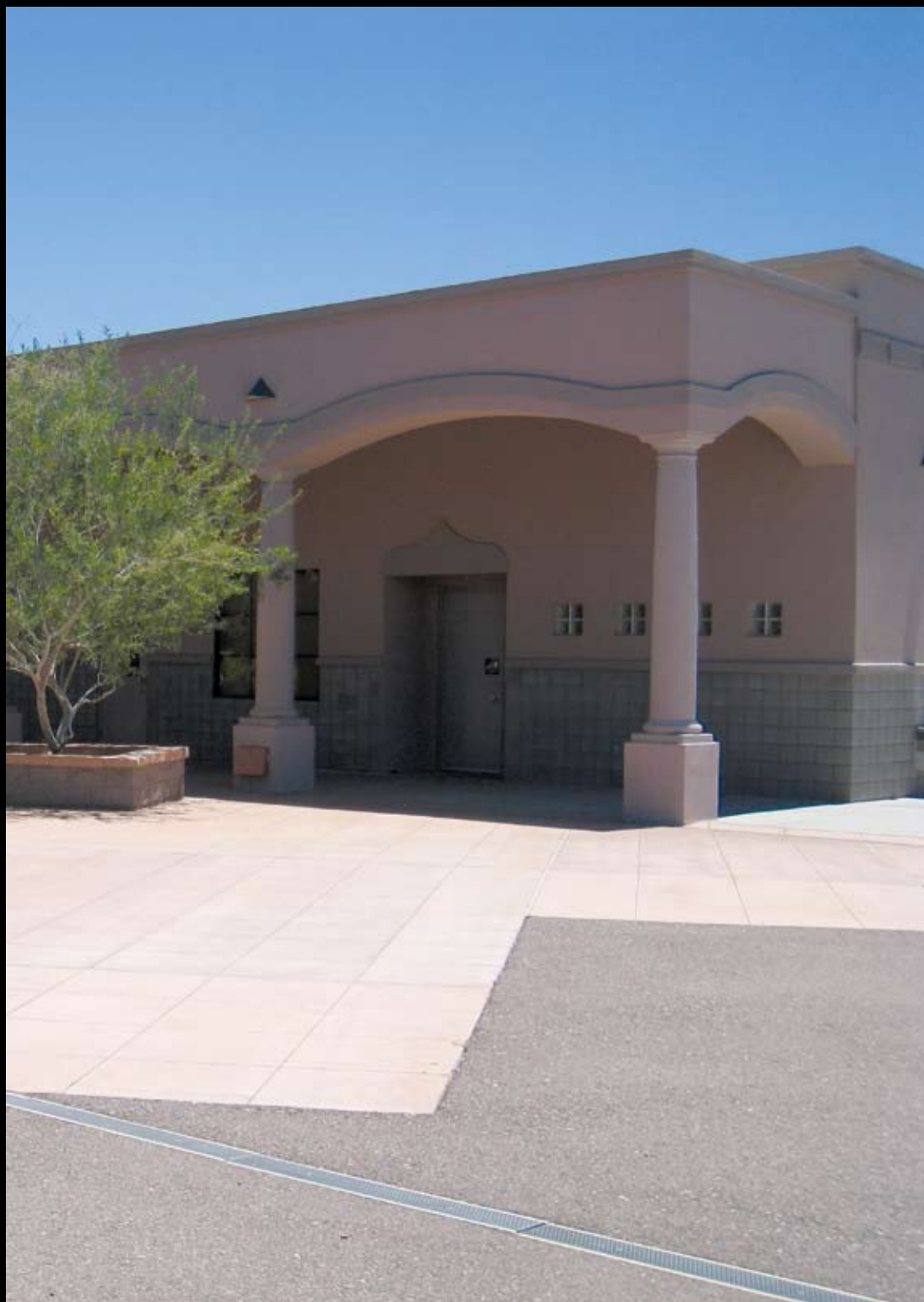
Interior courtyard in the Islamic Center of the Northeast Valley, Scottsdale, Arizona.
