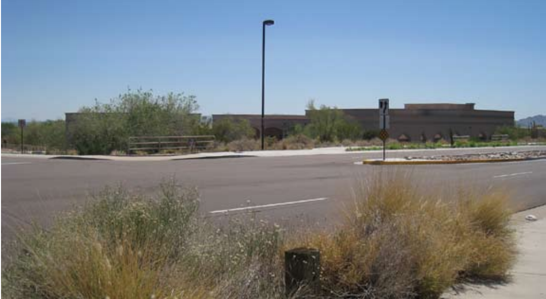
Mosque structure in Scottsdale, Arizona reflects design compromises.
